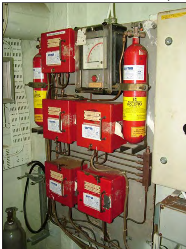
Master Control Unit (MCU) panel on Deck 14
