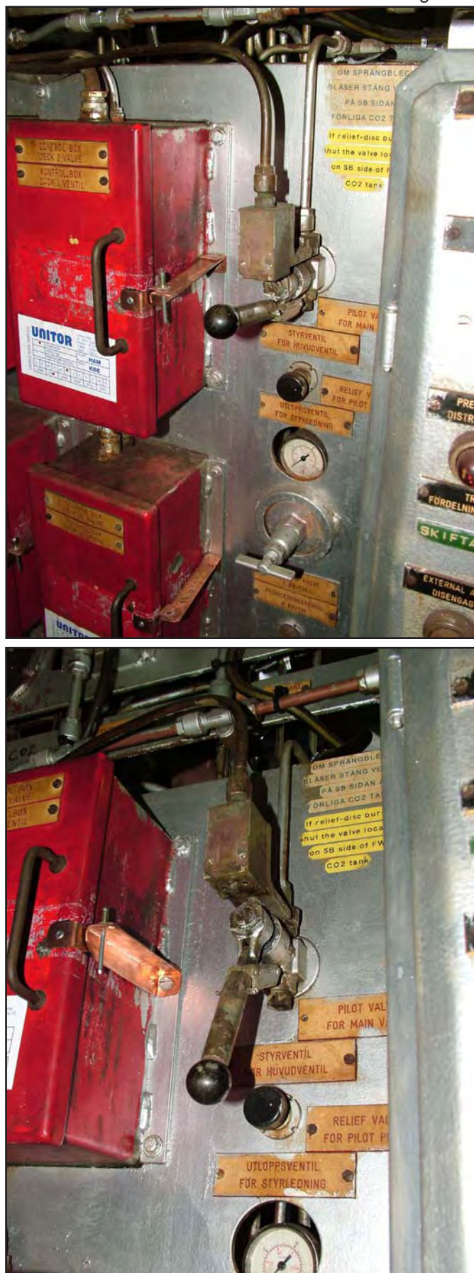
Main pilot release control valve on the CO 2 room control panel
